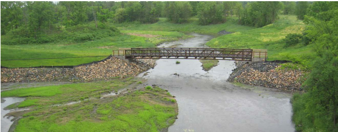
Figure 2. Woodley Dam Post-Removal (Same View as Figure 1).
