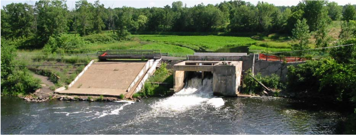
Figure 1. Woodley Dam Pre-Removal (Powerhouse Already Removed).
