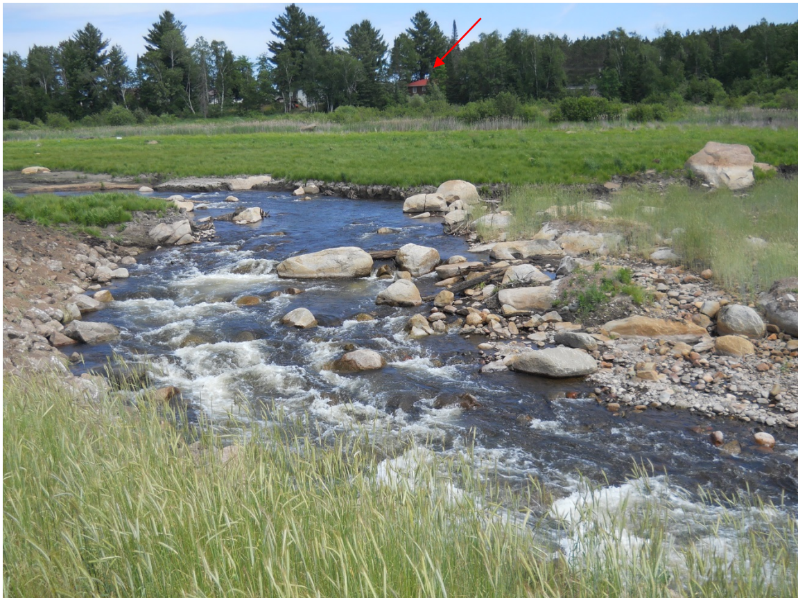
Figure 4. Grimh Dam Post-Removal.
